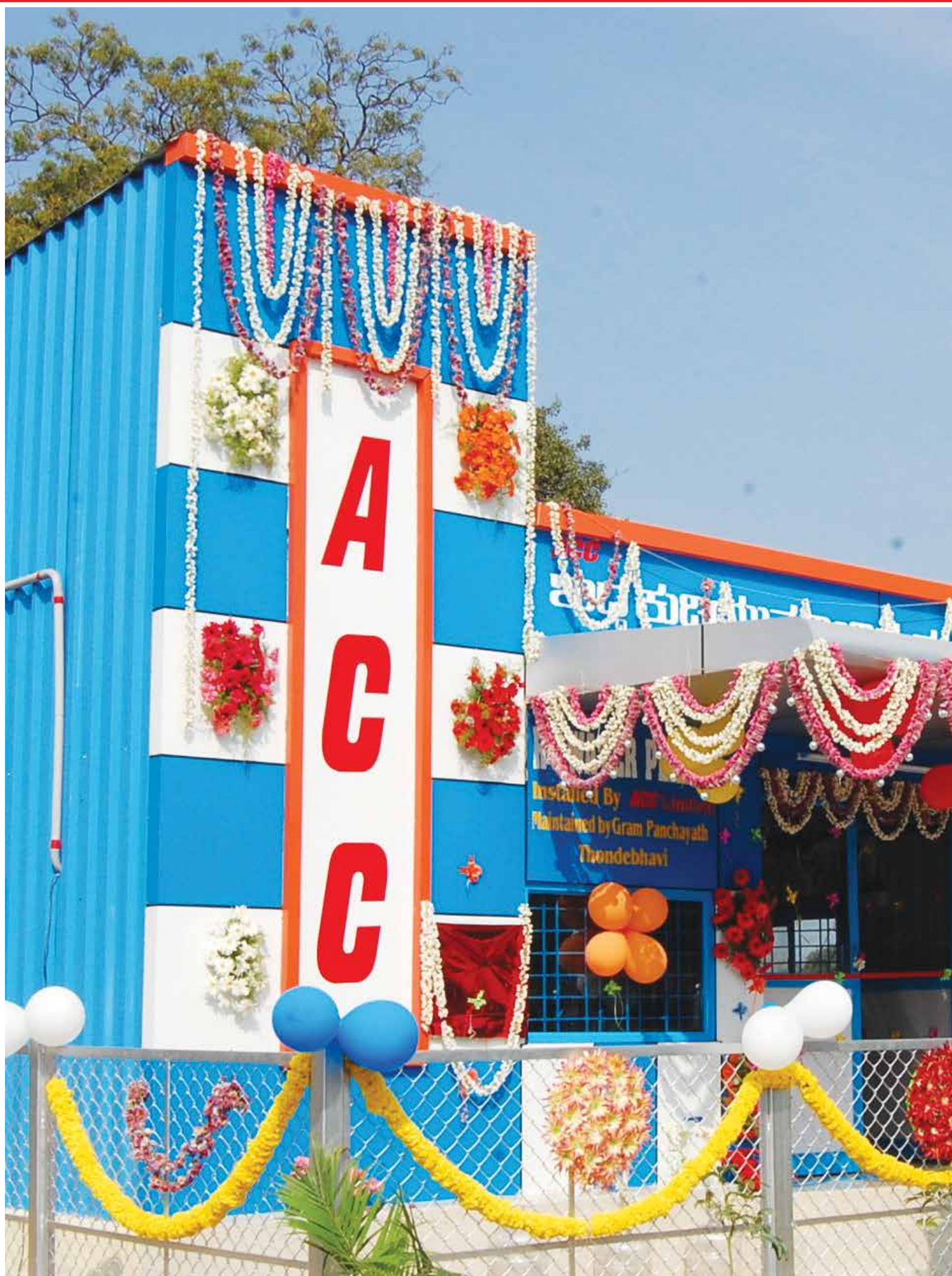
RO water plant installed at Thondebhavi village decorated for inauguration
