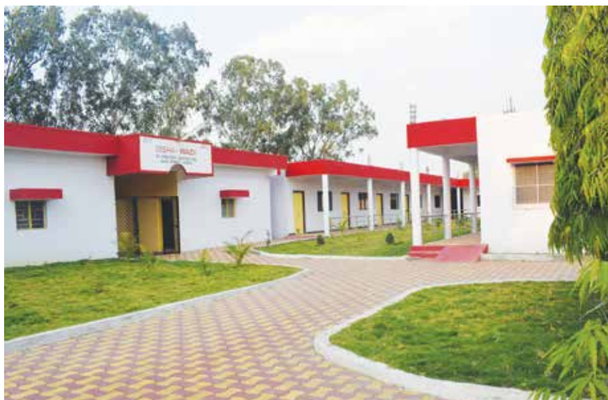
Newly constructed Alternate Livelihood Hub
